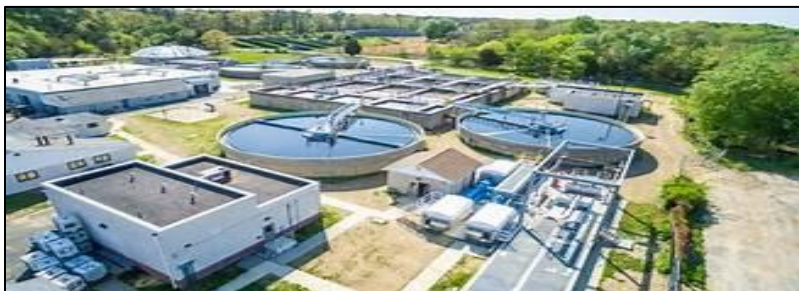
Fig. 5.5 Sewage Treatment Plant
