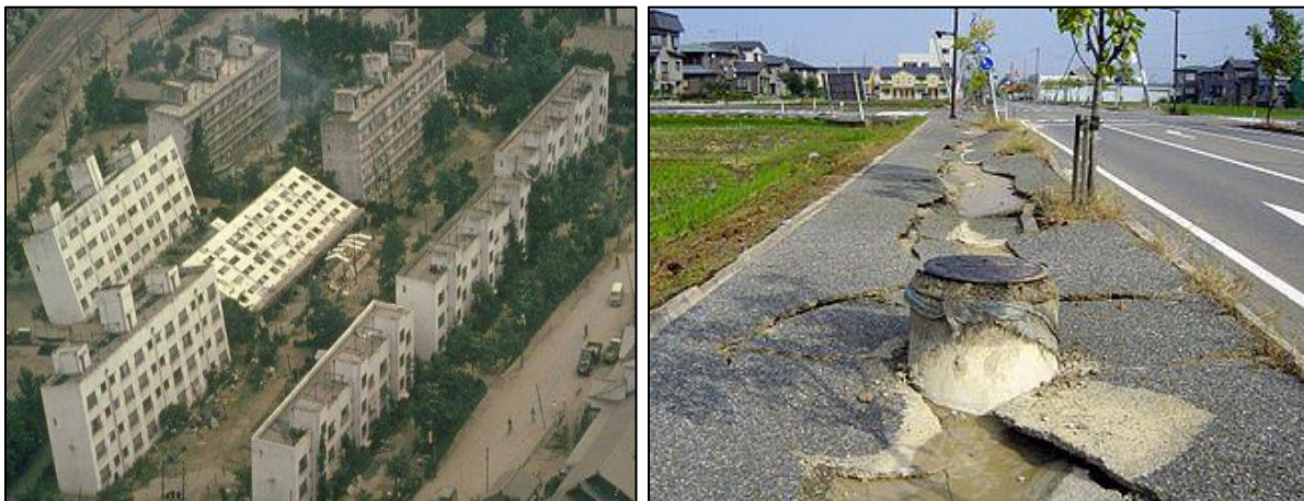
Fig. 5.1 Some effects of soil liquefaction
