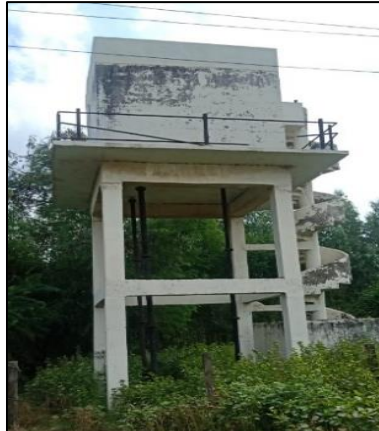
Fig. 4.5 Overhead water tank
