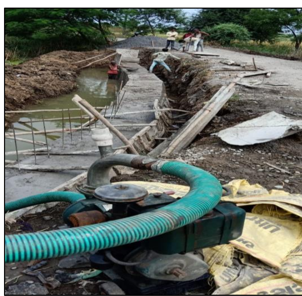
Fig. 12.17 Repair/Maintenance of Road
