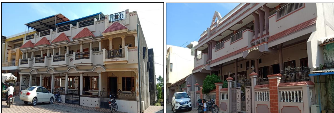
Fig. 12.3 Photos of Houses in Ena
